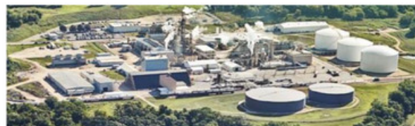
East Dubuque, Illinois Facility
